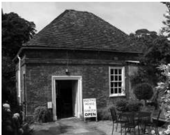
Wallingford Quaker Meeting House, built 1724
